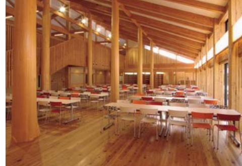
The Summit HR Construction System was used for a building at Kameyama Seki Junior High School in Mie using local cedar timber.
