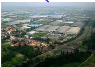
EJIP Industrial Park (contractors: around 100 site area : 320ha)
