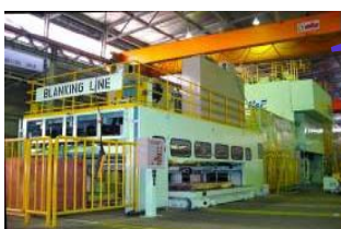
Steel Service Center (3plants, Production capacity : 420K MT/year)
