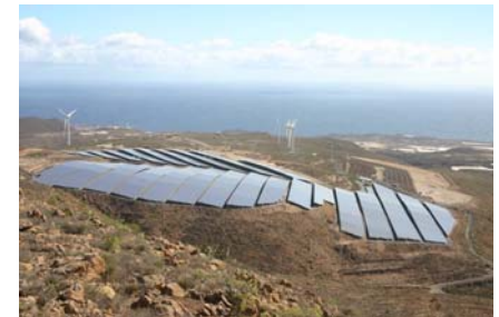
Solar power generation project in Spain
